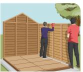
**O2** Building the walls Start with the back panel and place it on the base, but do not attach it to the base just yet. The panel with the door must be placed last, so keep this in mind as you build. Use a timber batten to keep the panels aligned if you unable to hold the panels in place.
