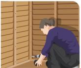
**06 Build then place** Only when the walls and roof are in place, physically attach the shed to the base. Ensure that it is square and correctly put together by using a spirit level on the edge of each panel. Use screws to attach the interior and exterior of the panels to the bases.
