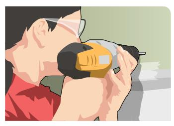
Where there's a drill there's a way You can use a standard drill bit for a stud wall, but you'll need a masonry bit if you're drilling into concrete. It will have to be a screw that's at least 30mm in length, so the easiest way to gauge this depth is to measure it on the drill bit and mark it with tape. Drill the holes slowly.
