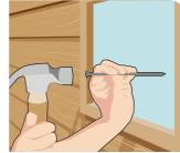
**03** Stabilise it Place a screw at the top, middle and bottom of the corner joint where the panels meet. It's advised to add screws into the bottom of the panels if your shed is bigger than average to stabilise it, but, for now, we need to use these screws to keep the panels level.
