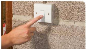
06 Let there be light! If you want to add any light switches, then we suggest that you run the negative feed straight through from the distribution block through to the actual light itself, but put the break on the live feed. Then, when you press down the light switch it'll turn on the light (hopefully, anyway). Just make sure that you buy a 12V lighting kit - and make sure that you use energy efficient bulbs, which could use just 22W per hour.
