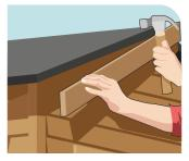
**OB** Finishing touches Your shed is nearly ready, but we recommend adding an end beam to the edges of your roof. They can provide extra cover for the felt against wind and rain. A thin beam of wood will work, so feel free to attach with nails or screws depending what you have to hand.
